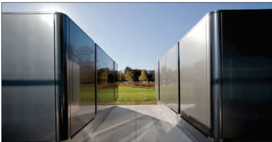
Two 100-kilowatt Bloom Energy Servers, as the company calls them, at a site in California.
